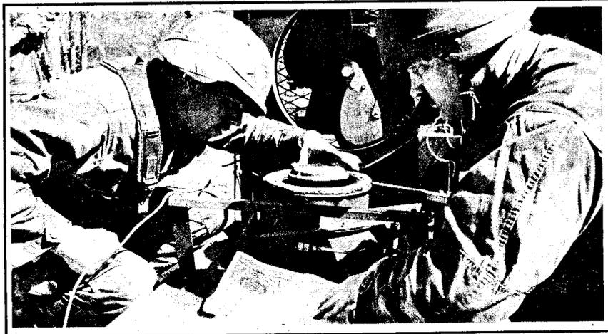
**BY THE BOOK** -- SP4 Terry Pevler (left) and SGT William Reed perform field repairs on a Herman Nelson heater during the 307th Maintenance Company bivouac at Pelham Range. Heater maintenance became critical when Alabama temperatures dropped into the teens.
