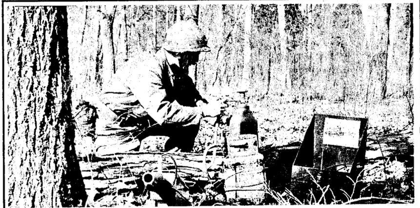
**GAS GUN** -- SP4 Roger Brooks of Elizabethtown checks out a machine gun simulator during field training exercises during last weekend's drill. The device utilizes liquid propane gas and a spark plug to simulate the sound of an M-60 machine gun. Assigned to the 35th Aviation Brigade of Frankfurt, Brooks said, "The training that we are doing today is as good as (that which) we get overseas." (Photo by SSG Ron Bayes, 133rd PAD)
